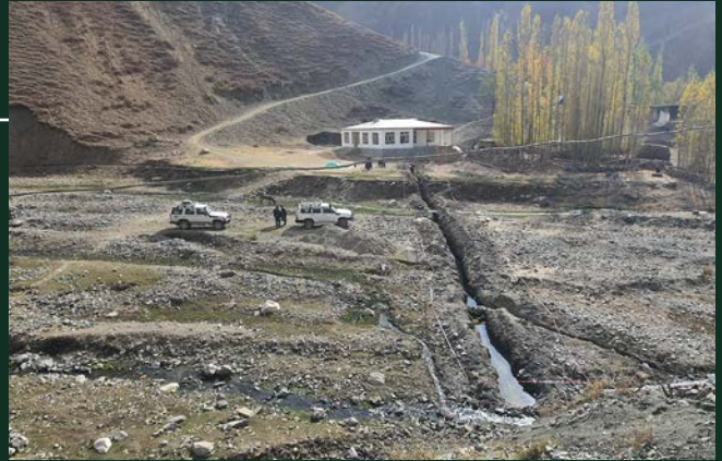
A water station under construction in rural Badakhshan Province, Afghanistan.
